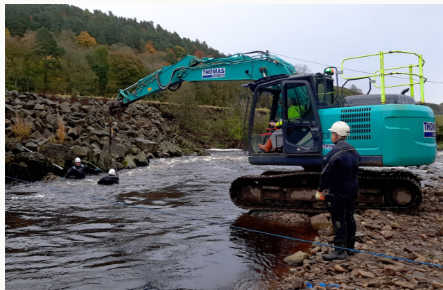
Pipeline inspection and maintenance works at River Allen crossing.
