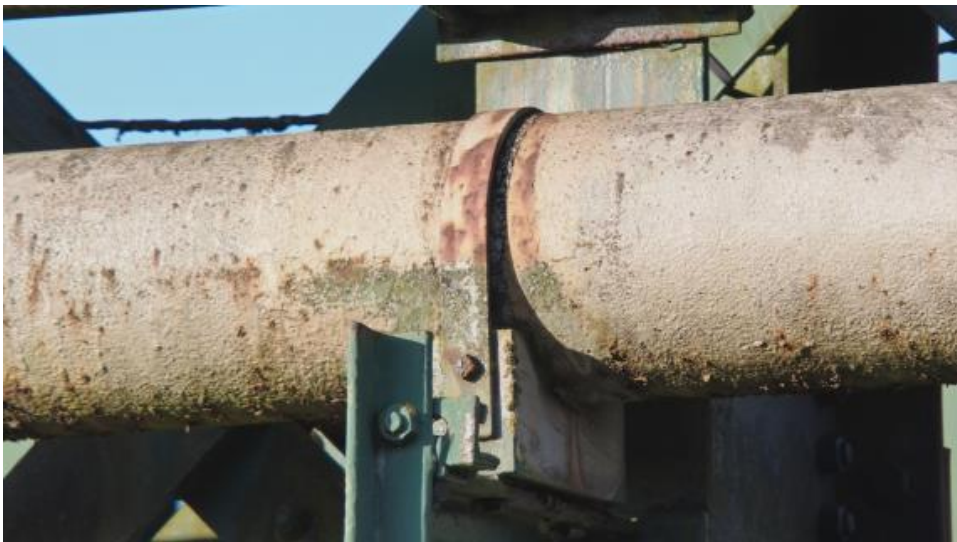
Figure 4 Drone imagery of one of the pipe supports
