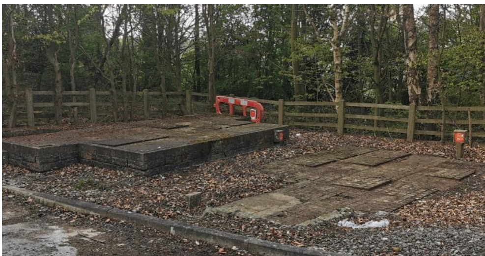
Figure 8 [REDACTED] Block Valve chambers before improvements
