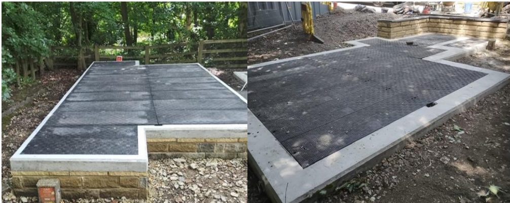
Figure 9 Block Valve chambers after improvements
