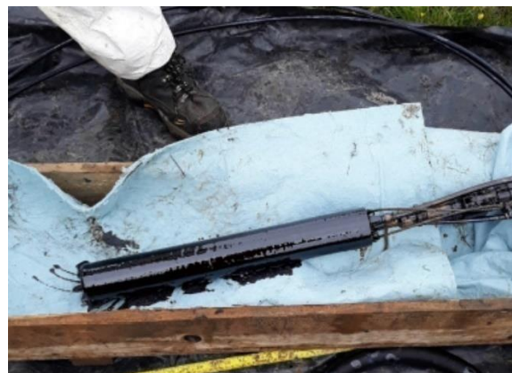
Figure 2 - Pump removed from a borehole for inspection and maintenance that was covered in viscous coal tar.
